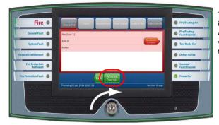
The fire control panel is operating in access level 2 when either Access level 2 or Key Level 2 is visible on the bottom-right of the touch screen display.
